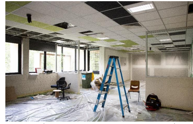
The HIVE (Health Immersive Virtual Education) Under construction
